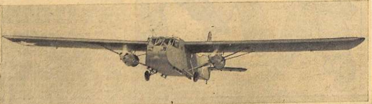
The Army's cargo and troop carrying gliders can now fly under their own power for short distances with the addition of two tiny engines shown mounted on this glider coming in for a landing at an airport in Minneapolis, Minn. Engineless gliders, similar to the one above, are now operating in the ETO with the Eighth Air Force Support Command.
