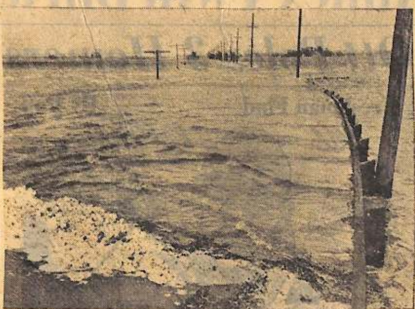
View of the highway from the east approach of Rocks Bridge, in the St. Louis flood belt, after the levee at Chouteau Island broke early in May, loosing Mississippi waters upon thousands of acres. It was called the worst Mississippi flood in 100 years, destroying millions of dollars worth of crops and washing out many homes.
