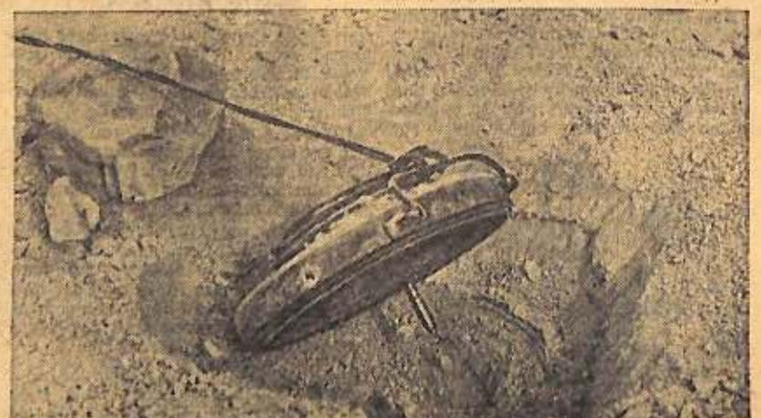
TELEPHONE WIRE, tied to buried mine, was one German trick. Canadian backs to safe distance before pulling wire to explode charge.
