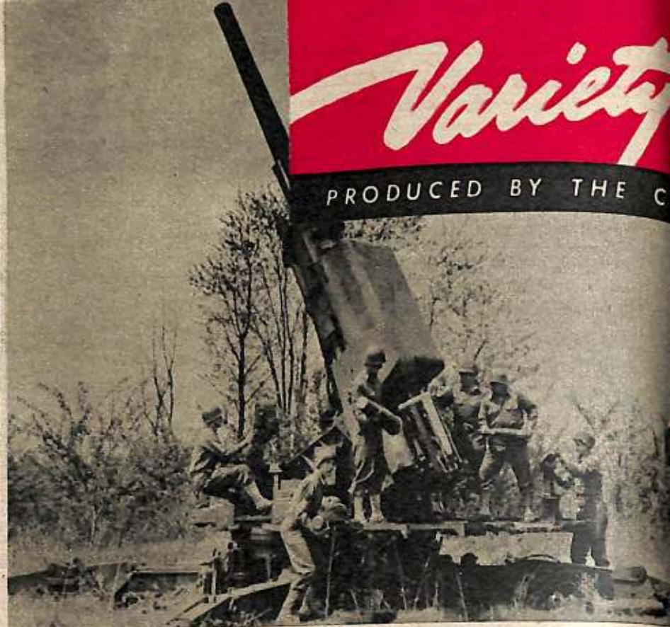
AIMING HIGH. Enemy altitude flyers beware. This U. S. Army 120-mm (4.7-inch) gun fires 20,000 feet higher than any other antiaircraft weapon in the world.
