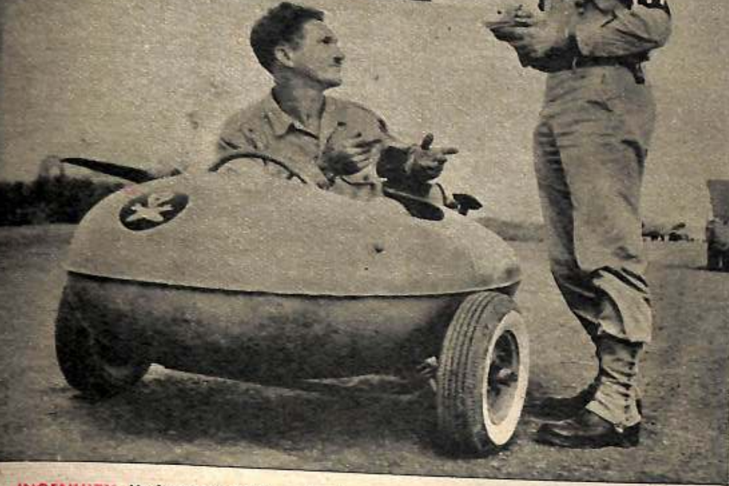
INGENUITY. He hates to walk, so in New Guinea Sgt. Maurice Tombaugh, Minden, Nebr., tells T-5 John Openshaw how he made a car mainly from plane's belly tank.
