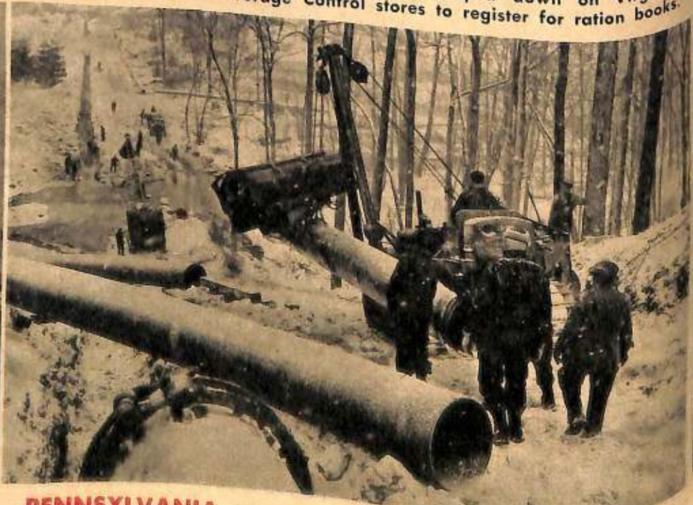
PENNSYLVANIA. Workers lay the world's largest pipe line which will carry oil for 1,388 miles when completed, from Texas to New York.
